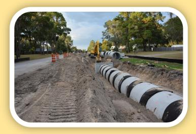
To construct the drainage pipes located under the roadway, the existing two travel lanes will be shifted to the southern right of way line. Two lanes of traffic will be maintained at all times.
